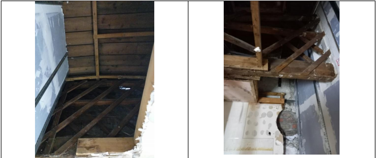
Figs. 4 & 5: View of Belfast Truss supporting curved roof.
